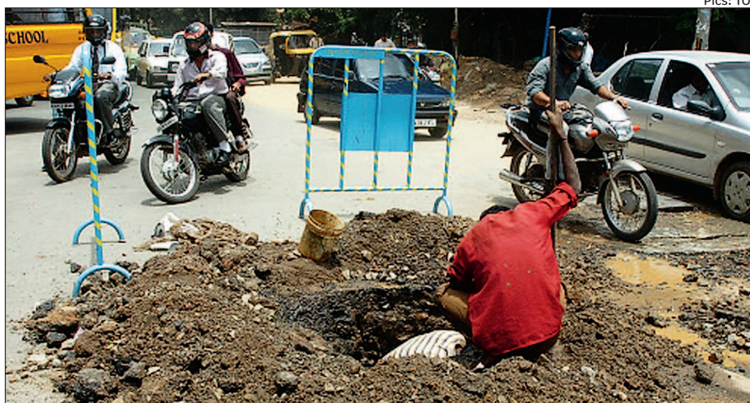
ROAD RAGE: Citizens are put to inconvenience because these critical civic agencies simply don't talk to each other
